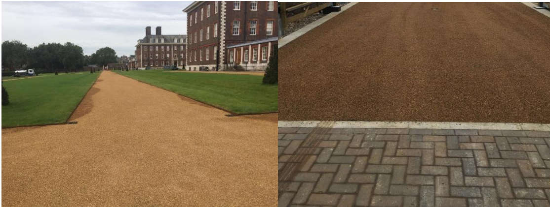
Figure 2: Surface Dressing - (Source: Foster Contracting)
